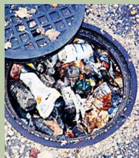
A trash-clogged combined sewer system can cause sewer backups and local flooding.
