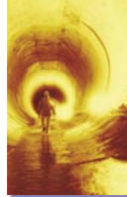
CSO underground tunnels will be equivalent to a 10-mile long subway tunnel, 25 feet in diameter.
