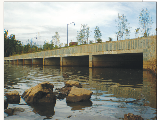
Completed overflow and diversion structures
