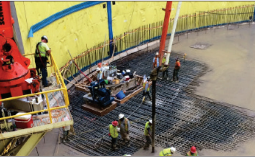
Base slab construction at Blue Plains Tunnel shaft
