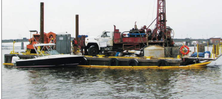
Drilling rigs on the Anacostia River take soil borings.
