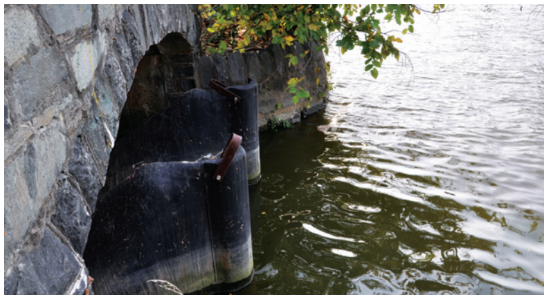
One of 15 CSO outfalls on the Anacostia River
