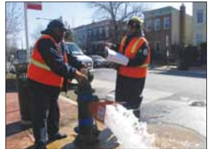
program and a temporary switch in water disinfection are conducted to enhance drinking water quality and minimize the impacts of aging pipes. The average age of a water main in the District is 78 years old.
