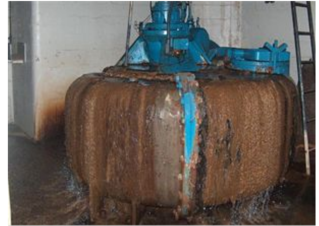
Failed Stormwater Pumps
