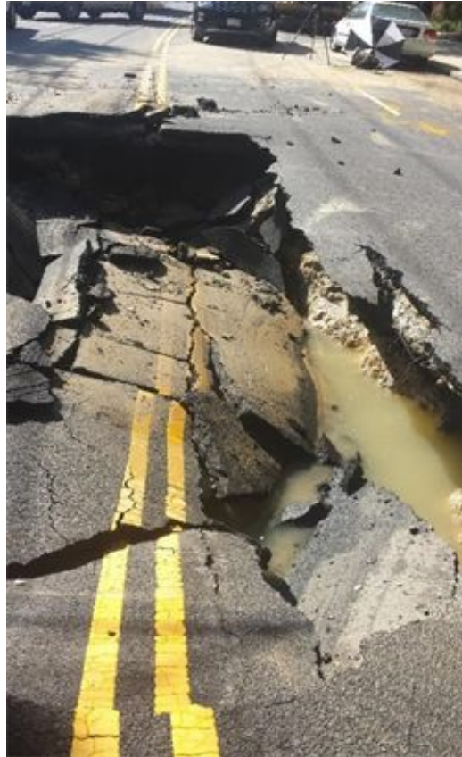
Q St. NW Rupture of 30" cast iron pipe c1860,
