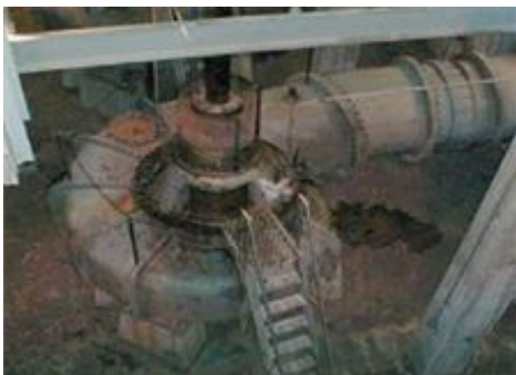
RWWPS I Worn out Pump
