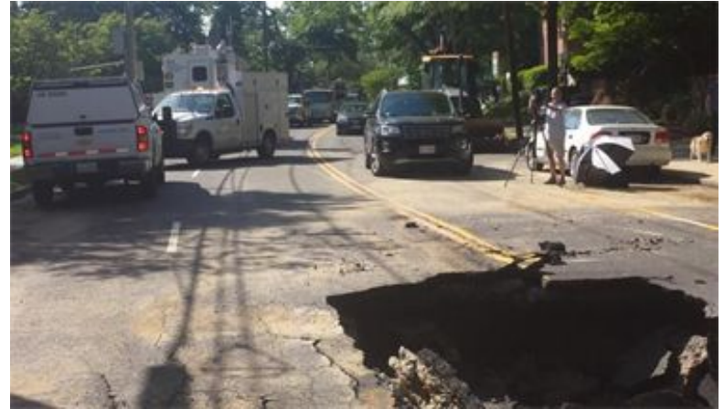
Q St. NW Rupture of 30" cast iron pipe c1860,
