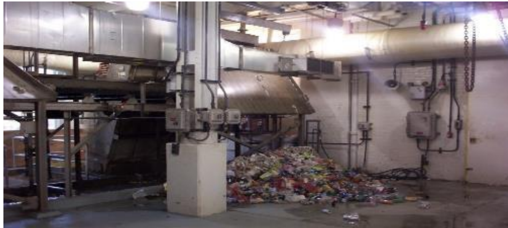
Lack of conveyance, washing and compacting
