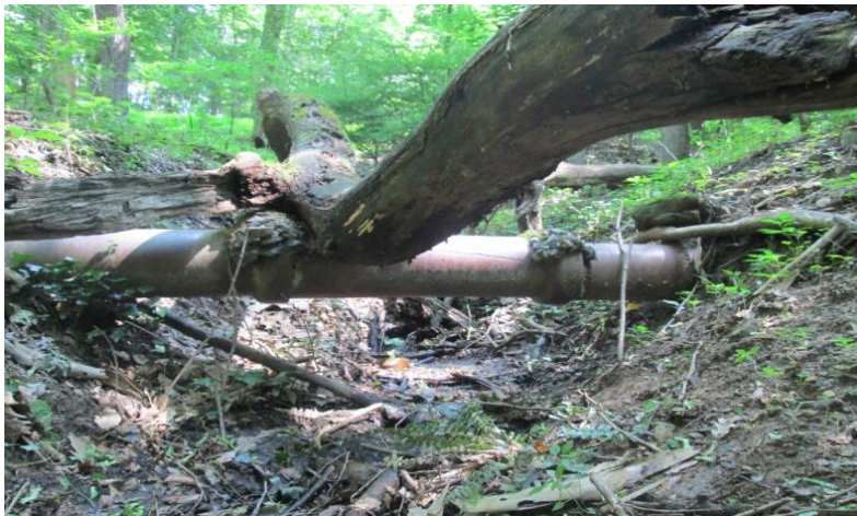
10" VCP Sewer pipe, installed in 1914, near Morrow Dr NW, located in Rock Creek Park.
