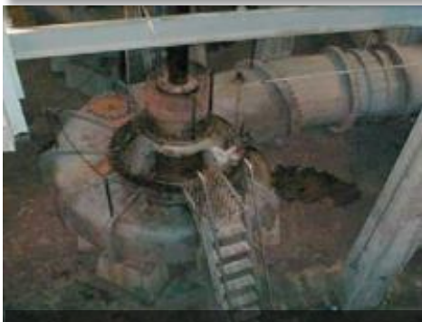
RWWPS 1 Worn out Pump
