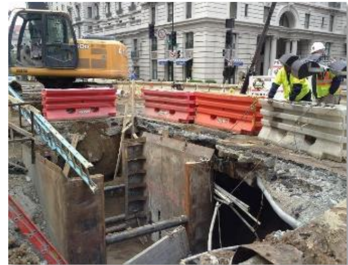
Q St. NW Rupture of 30" cast iron pipe c1860,
