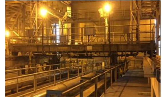
Screens, Grit & Primary Facilities Upgrades
