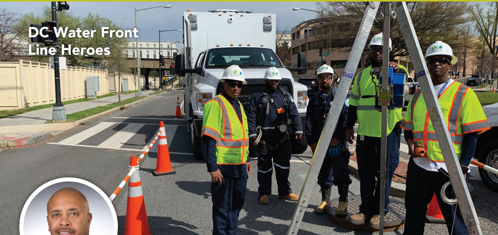
DC Water's elite SAM 101 team prepares to inspect a CSO-prevention inflatable dam in the sewer system
