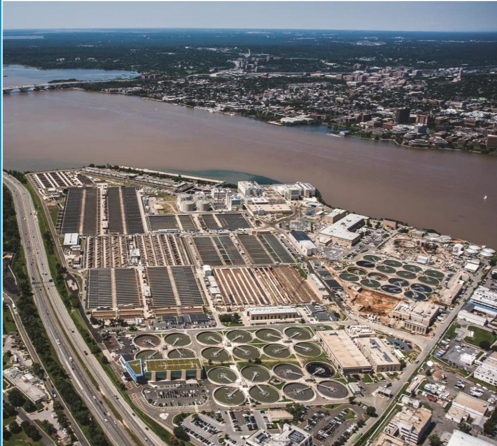
Blue Plains Advanced Wastewater Treatment Plant
