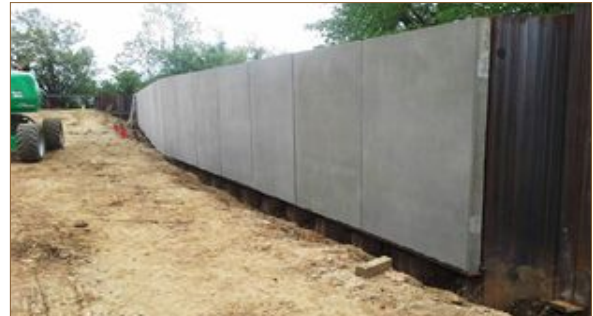
Blue Plains floodwall installation
