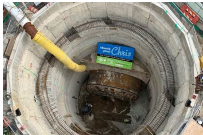
Tunnel Boring Machine "Chris"
