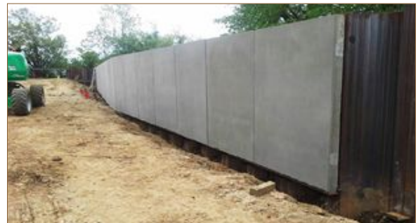
Blue Plains floodwall installation
