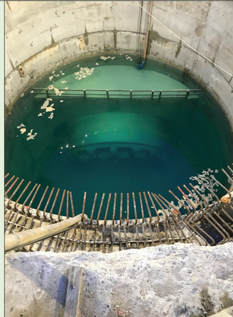
Above: The TBM cutterhead breaks through the concrete shaft, as seen from above and under water. Outside Flap: After finishing his five-mile journey, TBM Chris rests before getting a lift out.
