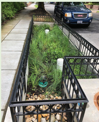
(l) Bioretention uses rainwater to sustain plant life, while filtering excess water through rocks into the ground. (r) Alley constructed with pavers that soak up the rain.
