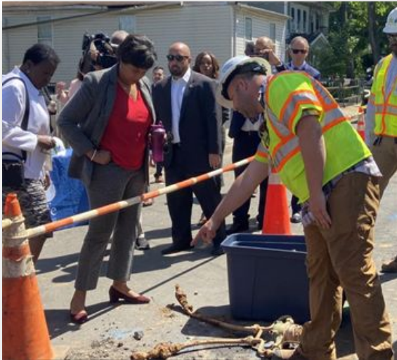
Mayor Bowser at Ward 7 Block-By-Block replacement.
