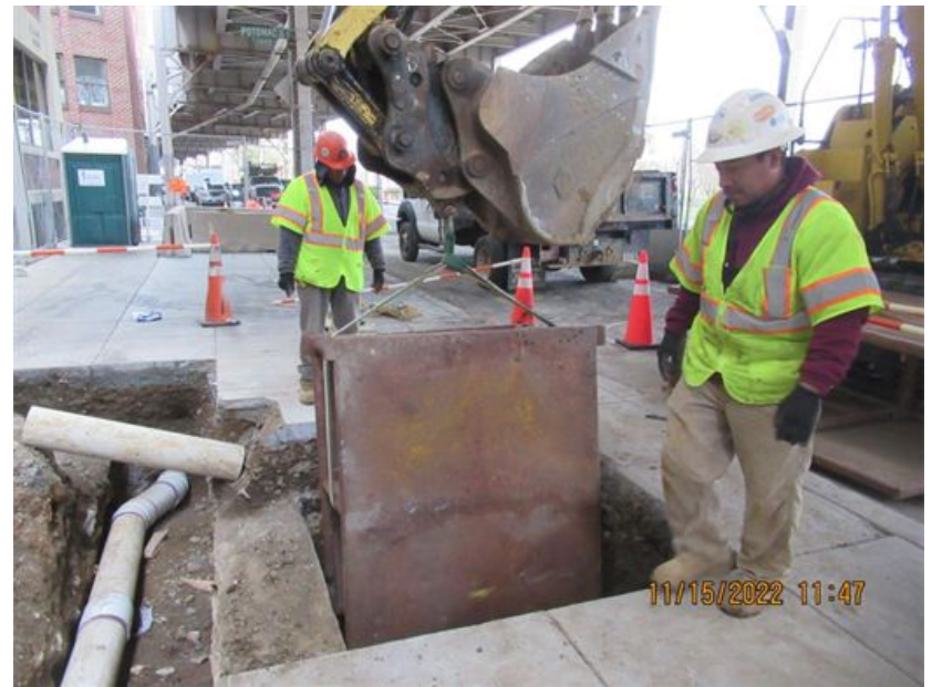
Test Pitting Activities at Structure 44
