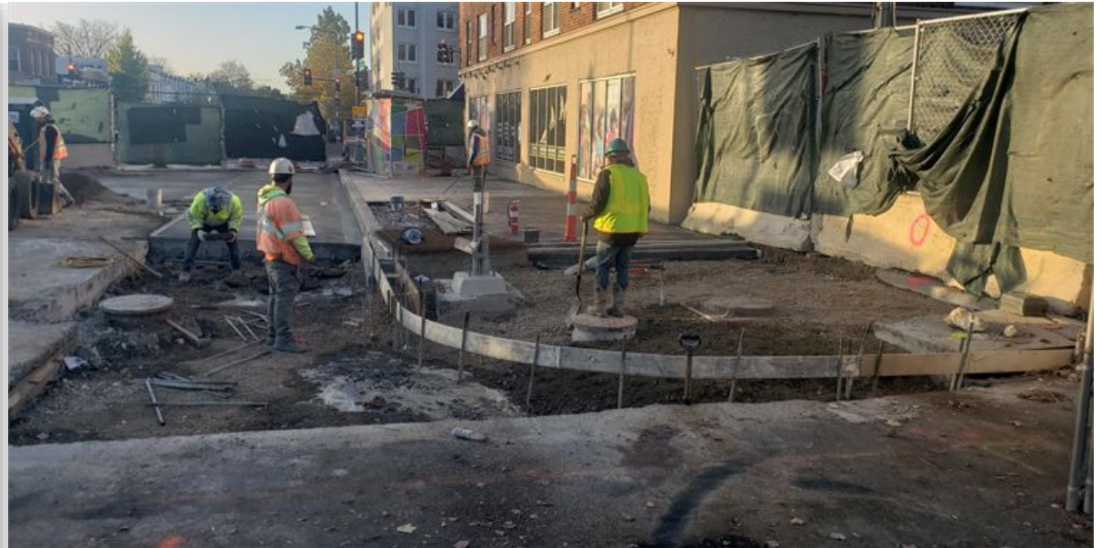
4 th Street Restoration
