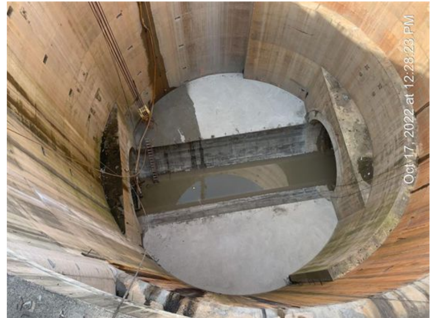
North Shaft Invert
