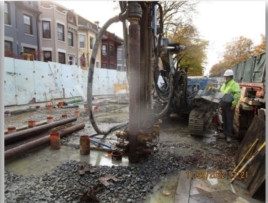
Construction Staging Area 3 Micro Pile Installation
