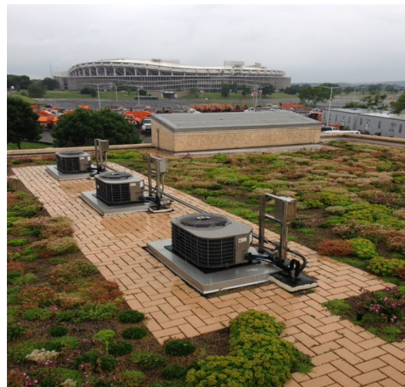
East Side Pump Station – Green Roof
