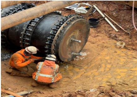
Soldier's Home Reservoir Upgrades
