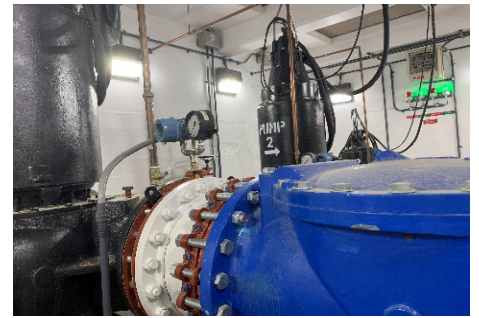
Stormwater Catch Basin
