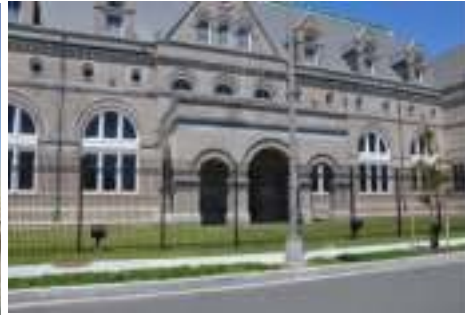
Bryant Street Pump Station
