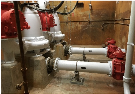
City Street Catch Basin
