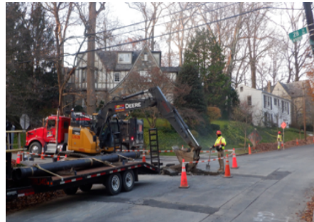
Small Diameter Water Main Repair
