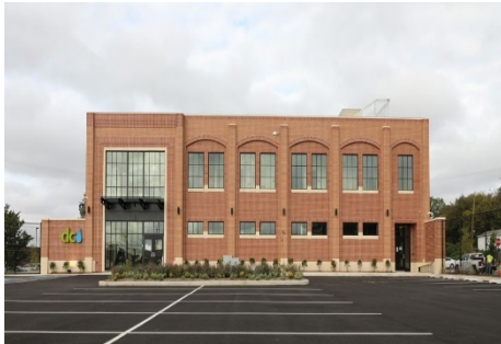
Non Process Facilities Sewer Building
