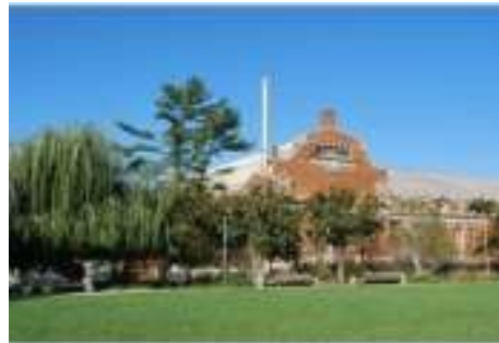
Main Pumping Station
