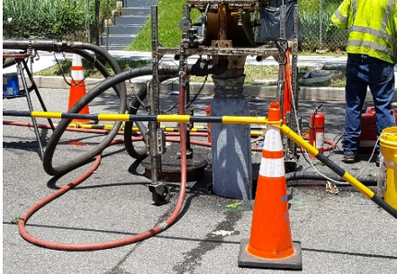
Sewer Rehab (Watts Branch)
