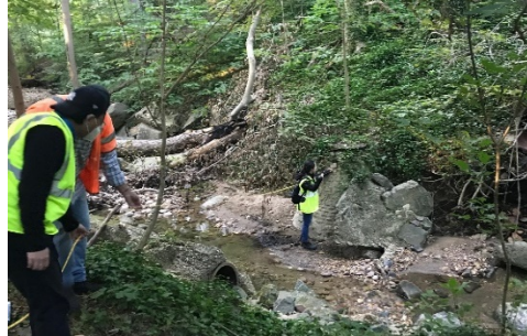
Rock Creek Stem Sewers (Condition Assessment)
