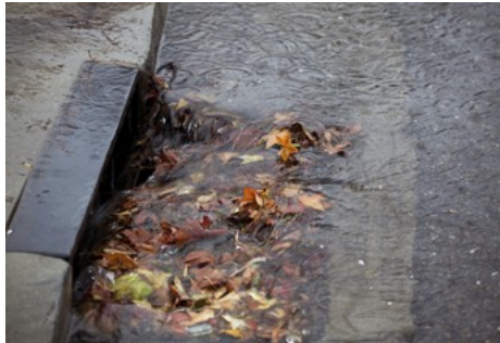
City Street Catch Basin
