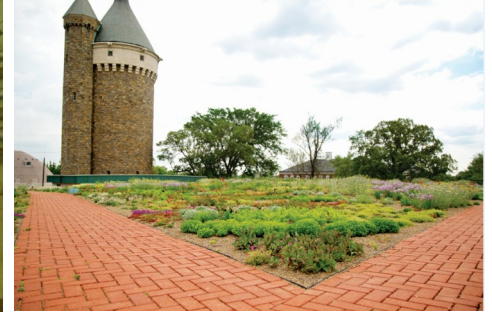
Fort Reno Green Infrastructure
