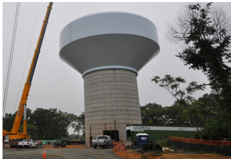
St. Elizabeth Water Tower
