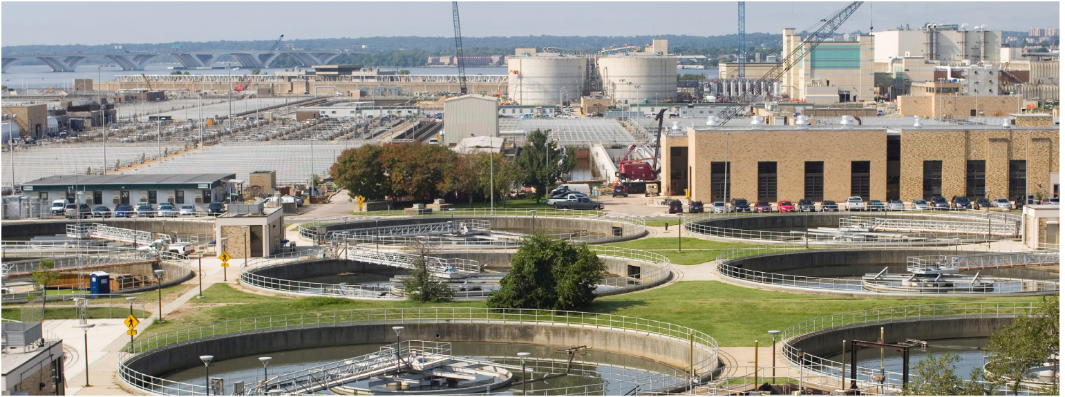
Blue Plains Advanced Wastewater Treatment Plant
