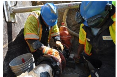
Water Meter Installation
