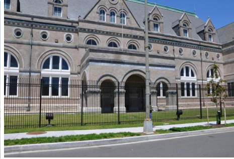
Bryant Street Pump Station
