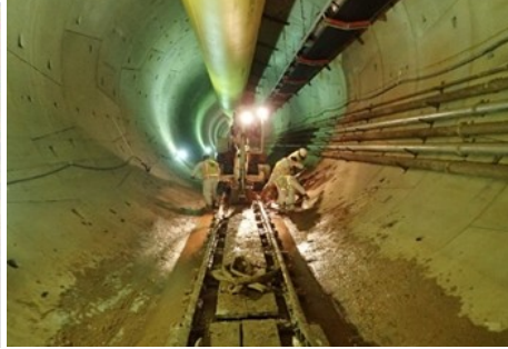
Northeast Boundary Tunnel
