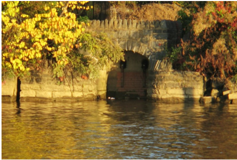
Combined Sewer Overflow Outfall
