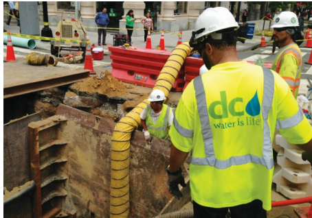
Sink Hole Rehabilitation
