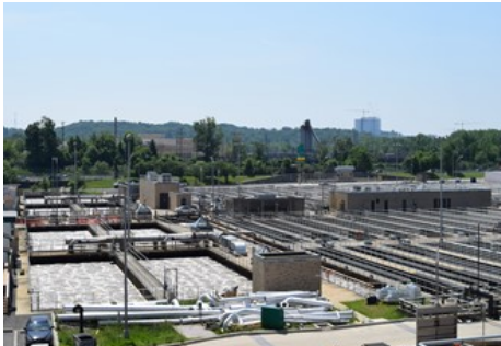
Blue Plains Advanced Wastewater Treatment Plant
