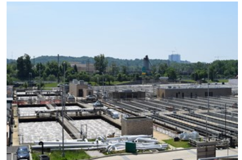
Nitrification Reactors
