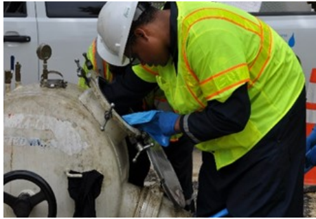
Sewer Line Rehabilitation Perma-liner
