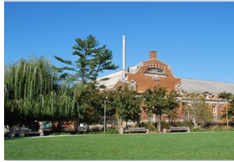
Main Pumping Station
