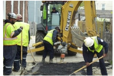
Linear Pipe Restoration
