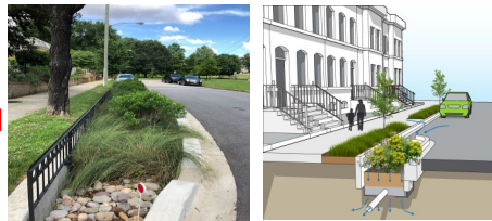
Curb Extension Bioretention (CBR)
