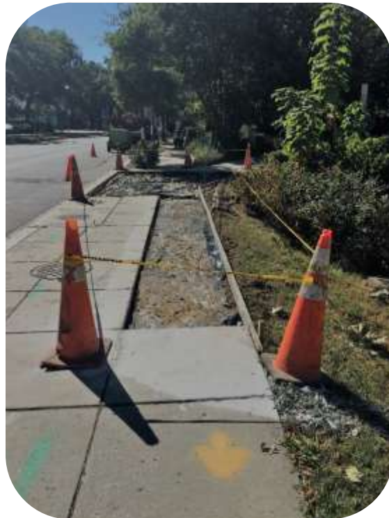
Figure 3: Repaving sidewalk on Rhode Island Avenue near T Street NW.
