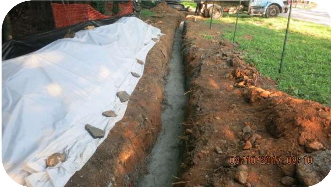
Figure 5: Trench for underground electric conduit.
