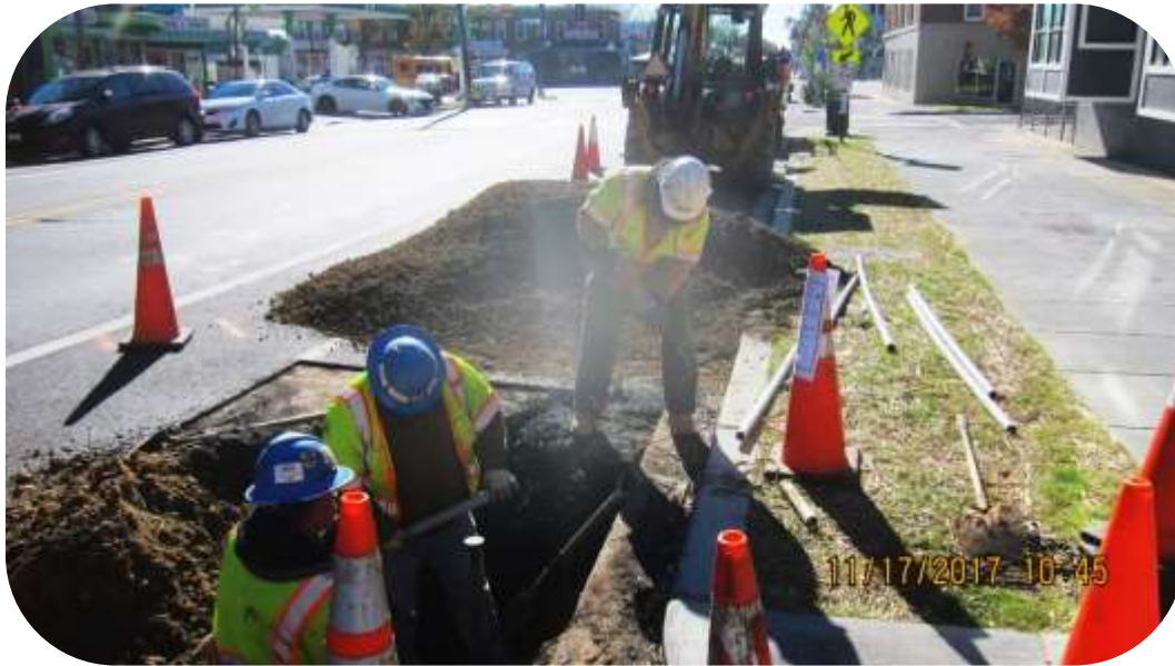
Figure 4: Installing MCI/Verizon Business conduit on 4th Street NE.
