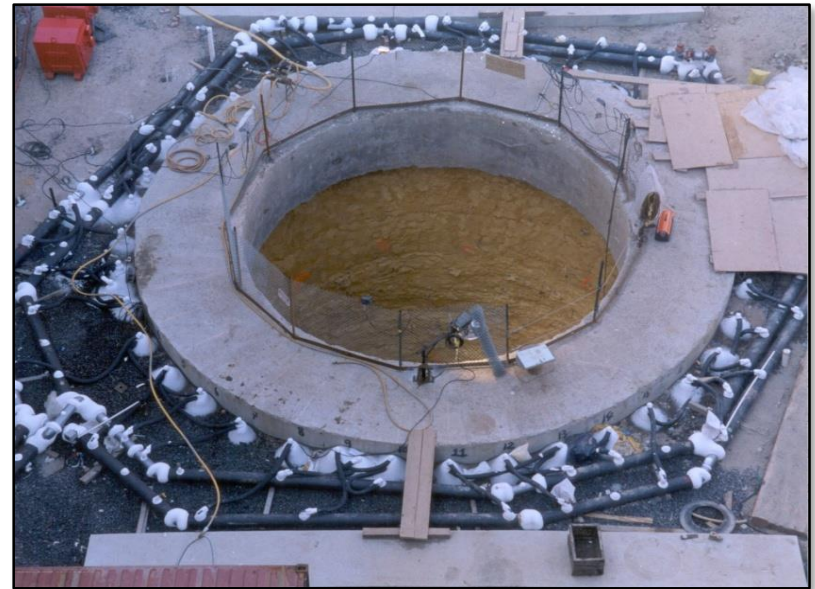
Example photograph of a shaft constructed using ground freezing
