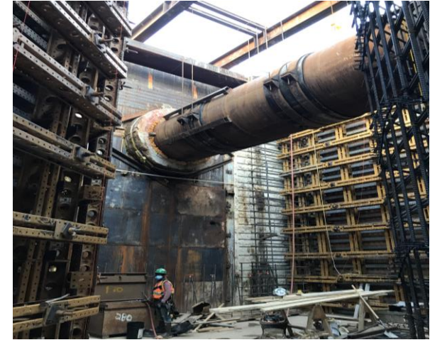
View of formwork for the diversion chamber and the temporary flume.
