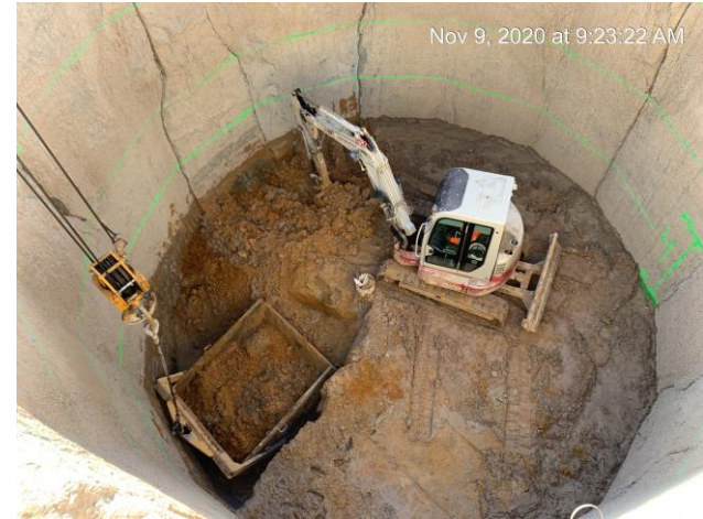
Excavating the drop shaft
