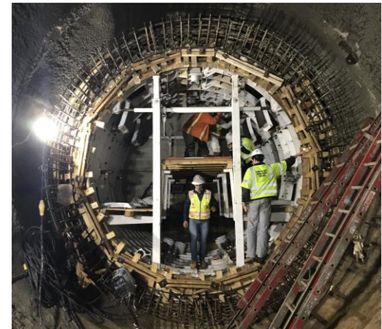
Lining the adit
