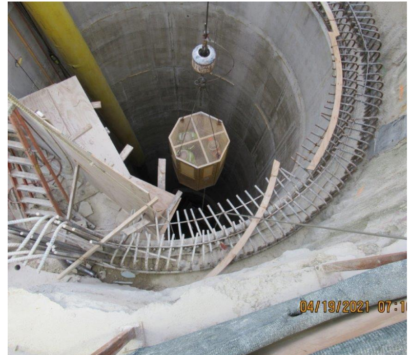
Inspecting the interior of the drop shaft.
