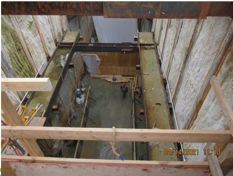
Setting forms for the approach channel base.
