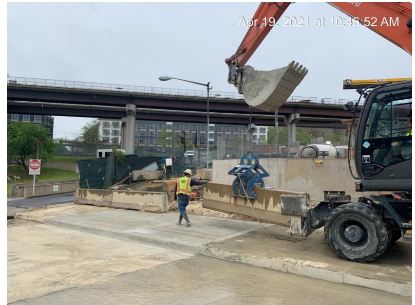
Lining the jersey barriers in preparation for changing the traffic pattern .
