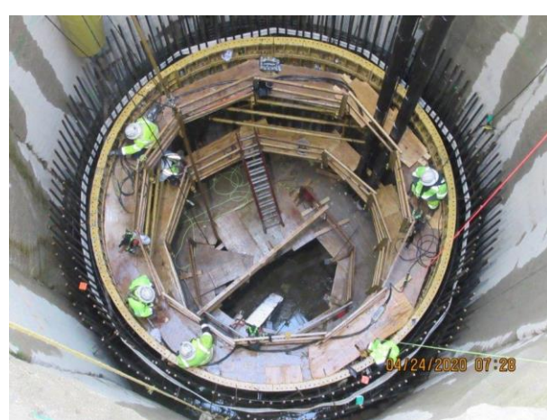
View down the drop shaft
