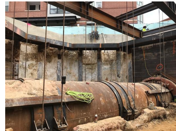
Flume serving as the temporary bypass of the existing sewer system
