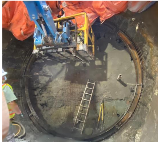
Excavating the adit
