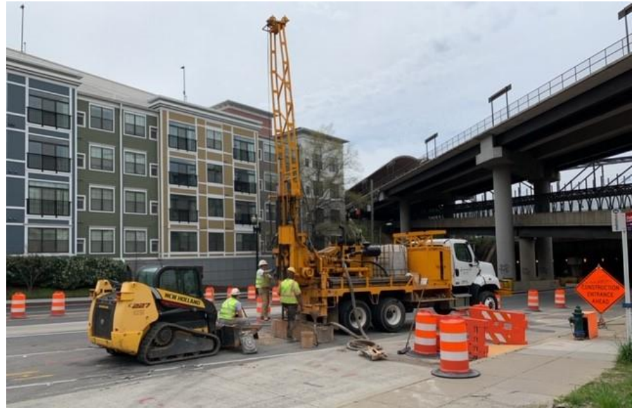
View of a Geotechnical Drill Rig
