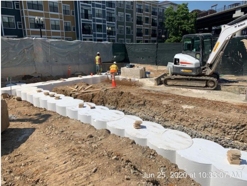
Setting secant guide wall formwork
