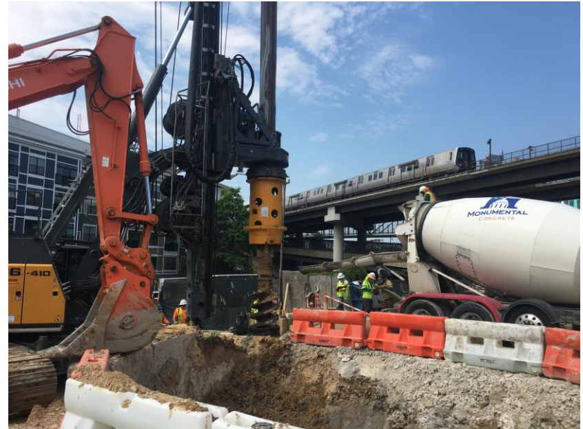
View of the drill rig used for installing secant piles
