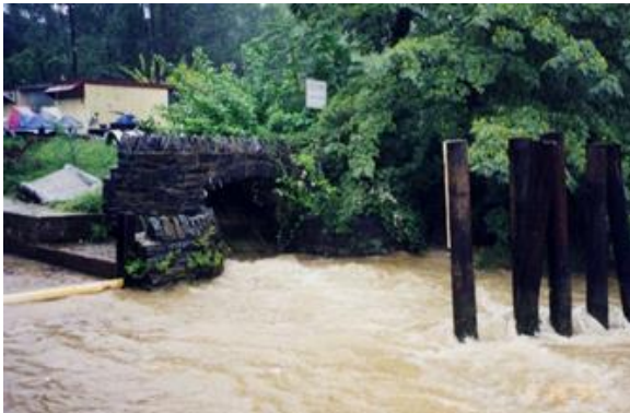
CSO Discharge to Anacostia River
