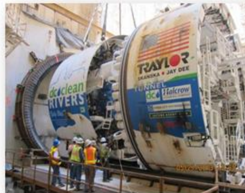
CHRIS, the Tunnel Boring Machine
