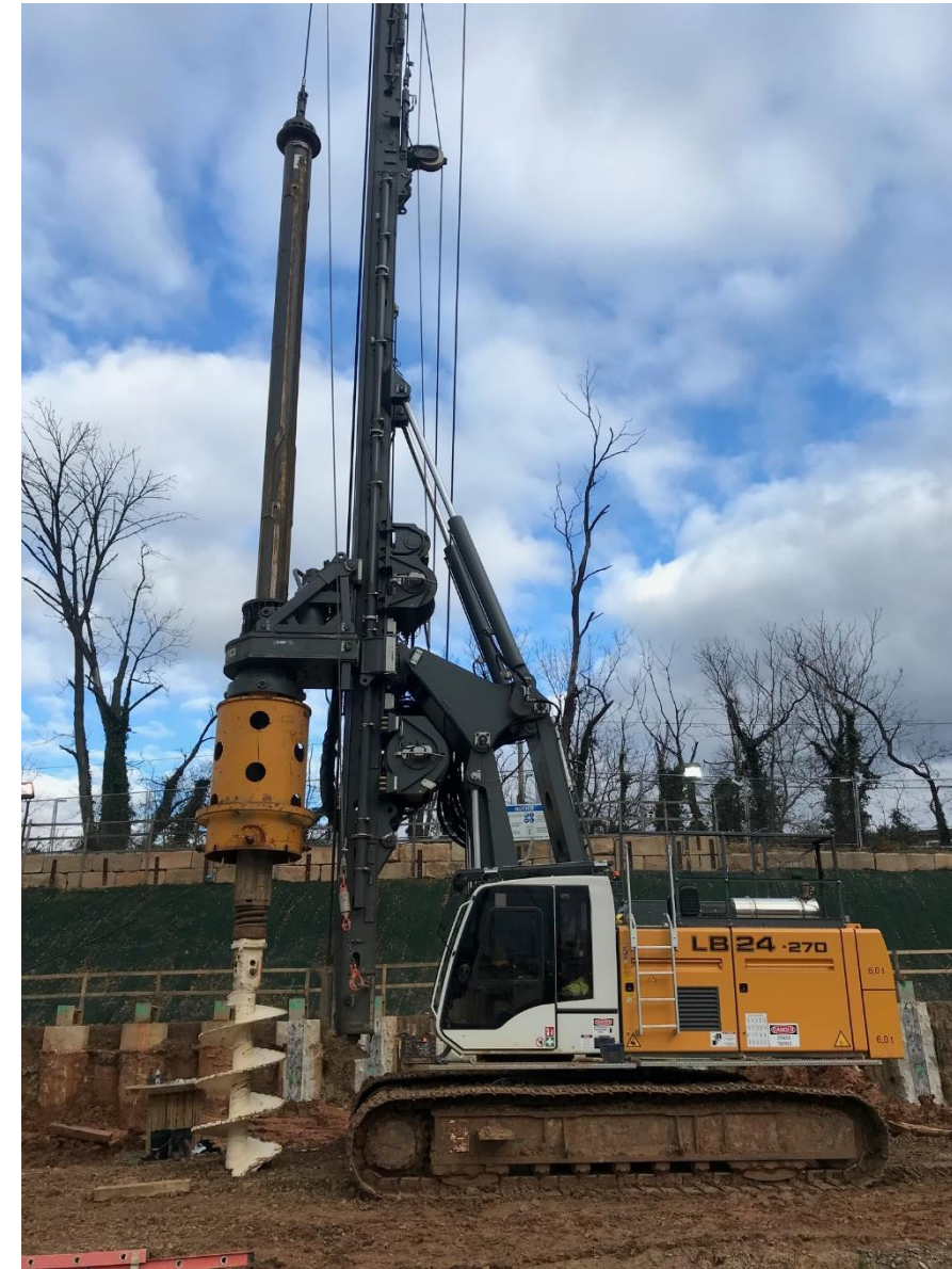
Caisson Drill Rig
