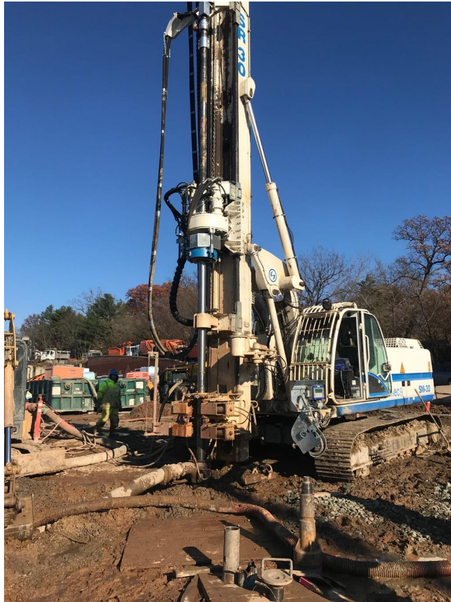
Jet Grout Rig
