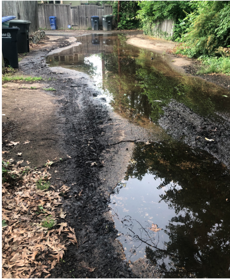
Exhibit 2 - Condition of Alley Grid 3195 taken during various times of the year.
